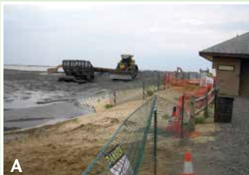
In July 2014, Bayshore Waterfront Park received 631,800 tons (390,000 cubic yards) of new sand, increasing the width of the beach from about 20 to 90 feet ( not including the new dunes). Photo A: Note the line between the older sand (right) and the incoming sand (left, darker grey color because it is wet.) B: The finished beach. C: By September, the wider beaches attracted swimmers, sunbathers, dog walkers and kayakers.
