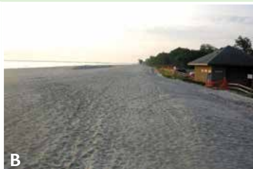
In July 2014, Bayshore Waterfront Park received 631,800 tons (390,000 cubic yards) of new sand, increasing the width of the beach from about 20 to 90 feet ( not including the new dunes). Photo A: Note the line between the older sand (right) and the incoming sand (left, darker grey color because it is wet.) B: The finished beach. C: By September, the wider beaches attracted swimmers, sunbathers, dog walkers and kayakers.
