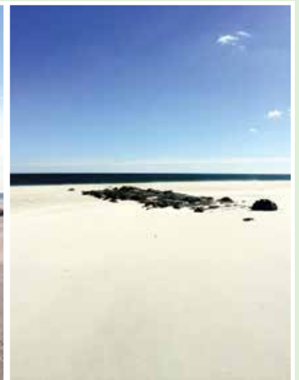
In February 2014, Seven Presidents received 409,860 tons (253,000 cubic yards) of new sand, increasing the width of the beach from about 180 to 410 feet. These photos show the same jetty at Kiernan beach, before and after replenishment.
