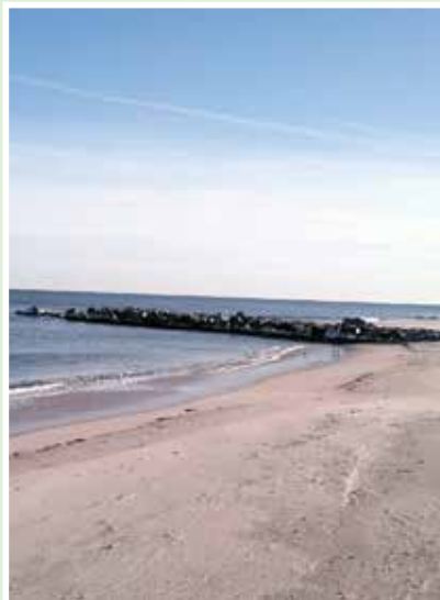
In February 2014, Seven Presidents received 409,860 tons (253,000 cubic yards) of new sand, increasing the width of the beach from about 180 to 410 feet. These photos show the same jetty at Kiernan beach, before and after replenishment.
